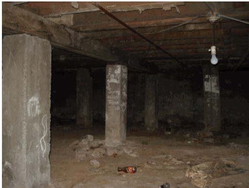
CONCRETE SUPPORTS IN CRAWL SPACE
