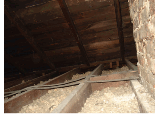
ATTIC INSULATION DEPTH TO VARRIED
